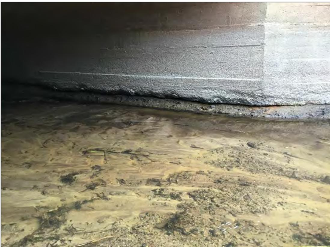
**Description: North abutment erosion at footing interface.**
