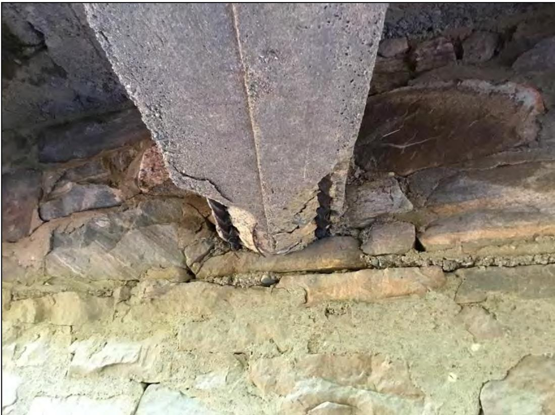
**Description: Exposed rebar on south side of east girder**
