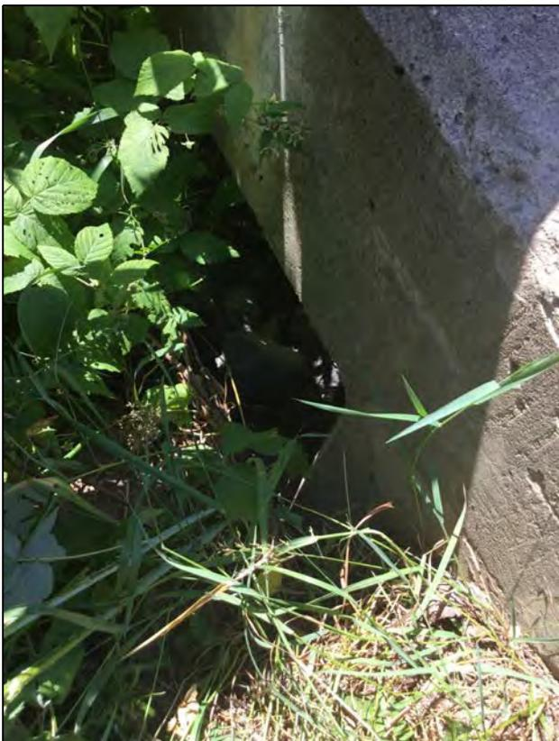
**Description: Eroded embankment at spillway southeast quadrant**
