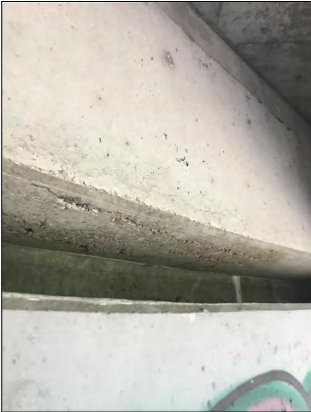
**Description: Scaling and delamination - north side third in Beams/Main Longitudinal Elements / Diaphragms (At north and south abutments.)**
