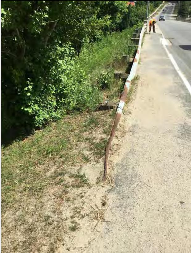
**Description: Bent NE steel beam guiderail**
