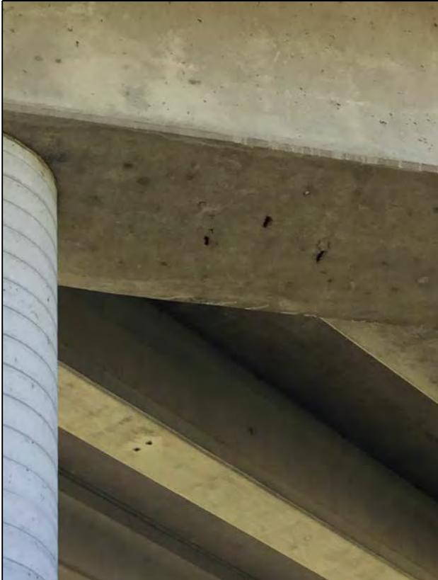
**Description: Minor spall w exposed rebar**
