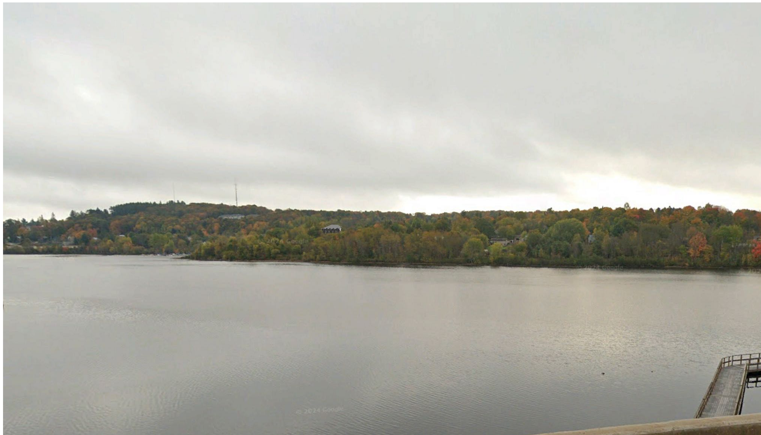
VIEW FROM HWY 11 BRIDGE
