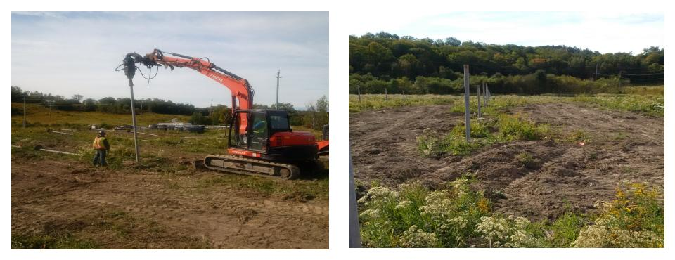
Helical pile installation and site grading work proceeded in summer 2019
